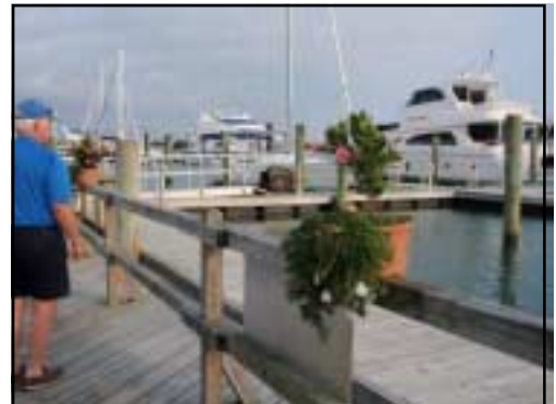
Carroll inspecting one of the harbors.
